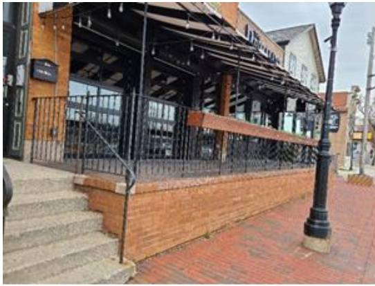
Existing Front Patio (Overall View)
